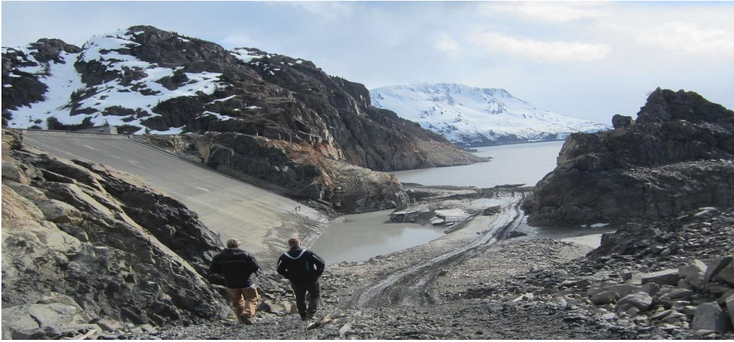
BRADLEY LAKE DAM, courtesy of Homer Electric Association, Inc.
